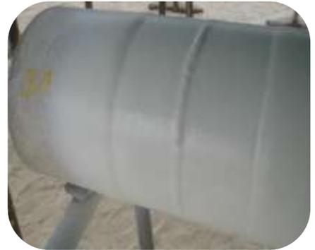
*Resichem 530 HA100 applied by brush to pipe field joints, while the coating was still wet Polypropylene was flame sprayed onto the surface of the Resichem 530 HA100.*
