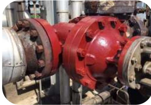
*As part of the site improvement plan over 300 valves , pumps and spools were coated Resichem 530 HA100. The coating was applied to surfaces operating at 150° C. Surface preparation was high pressure water jetting at 1000 psi to clean off any surface contaminants and the coating was applied at 300 microns per coat.*
