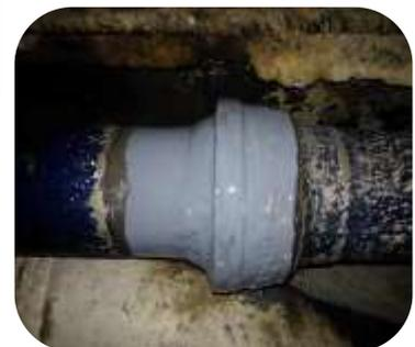
*Leaking pipe sockets on a diesel pipeline at a European oil refinery wrapped and sealed using 104 Metal Repair Fluid XF*
