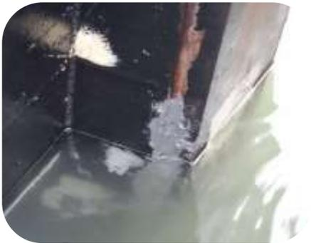
*Seal and rebuild damaged or worn surfaces underwater. 106 Metal Repair Paste XF can cure underwater at temperatures as low as 5° C*
