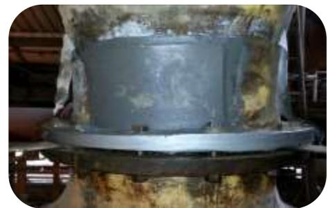
*Emergency repair to seal a leaking flange face on a cooler box*
