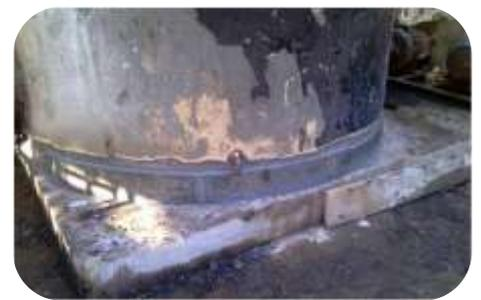
*Base of a chemical storage tank had been badly corroded from chemical attack. Surfaces were mechanically prepared using handheld grinders. A pre-formed steel plate was then bonded onto the damaged surface using 106 Metal Repair Paste XF .*
