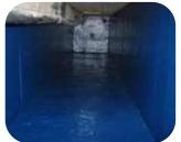
Resichem 573 Fastfill Screed is a single component fast curing engineering grade, polymer modified, reactive cementitious coating with high adhesive properties. It is used in permanent immersion or negative pressure waterproofing. It incorporates the most advanced micro-silica, polymer and fibre technology, curing to give a dense matrix which is impermeable to water under 10 bar hydrostatic head. Supplied as a single component system, ready for on-site mixing and use.
