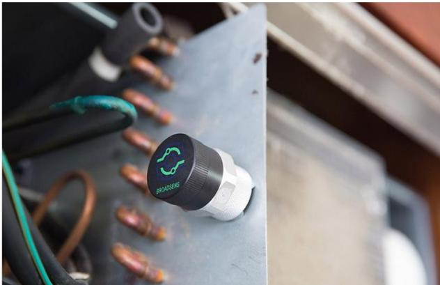
Wireless vibration sensor mounted on panel
